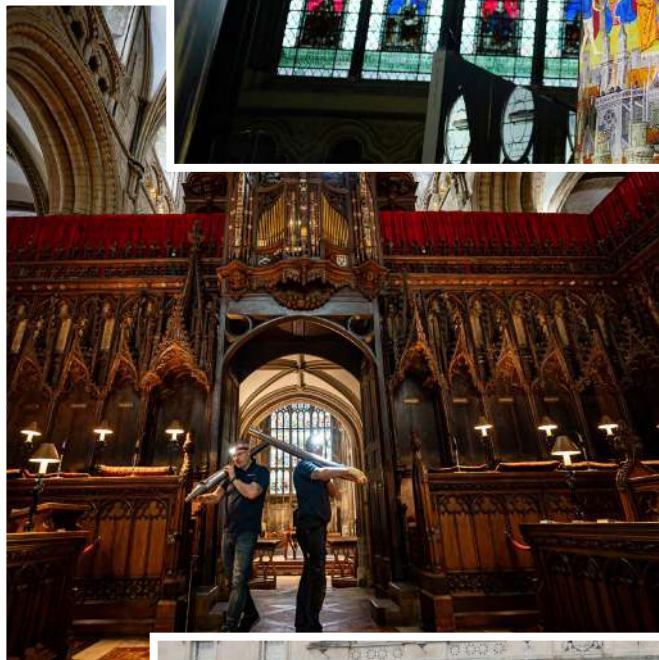
Specialists from Worcestershire organ builders Nicholson & Co Ltd remove and inspect pipes removed from the organ at Gloucester Cathedral, during its refurbishment in time for the 2026 Three Choirs Festival.
